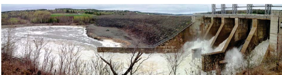
Figure Caption : 500 m long embankment dam and Diversion Sluiceway at Mactaquac Generating Station.
